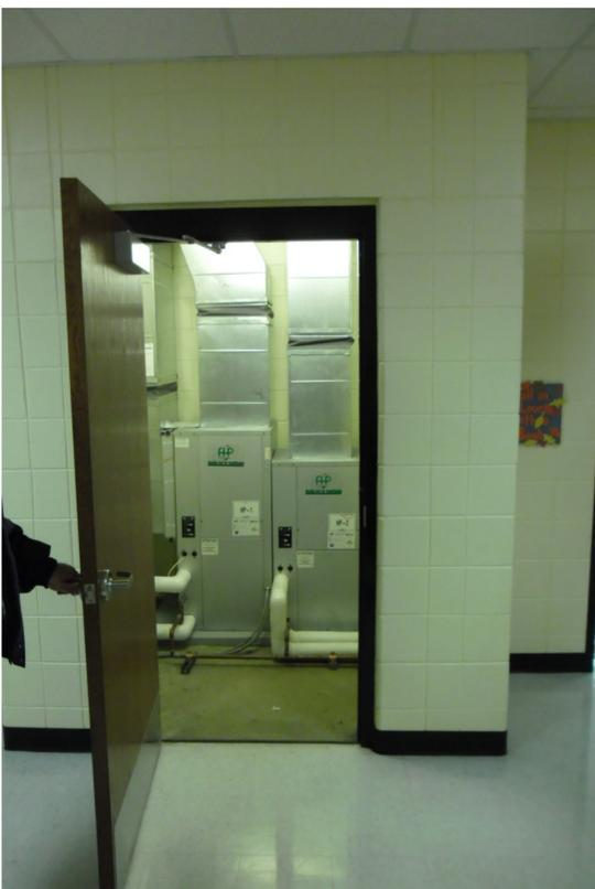
The Heat Pump Units are very similar to the heating/cooling unit at your home except that there is no gas burner and instead of the compressor being outside in a condensing unit, the compressor is inside the unit, similar to your refrigerator. When the unit is called upon to do cooling, cold refrigerant is sent to the air coil just as in your home unit, but when it is called on to do heating, the refrigerant cycle is reversed and hot refrigerant is sent to the air coil.
